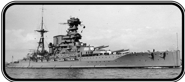
MASTRO ESTRUTURAL (STRUCTURAL MAST)
